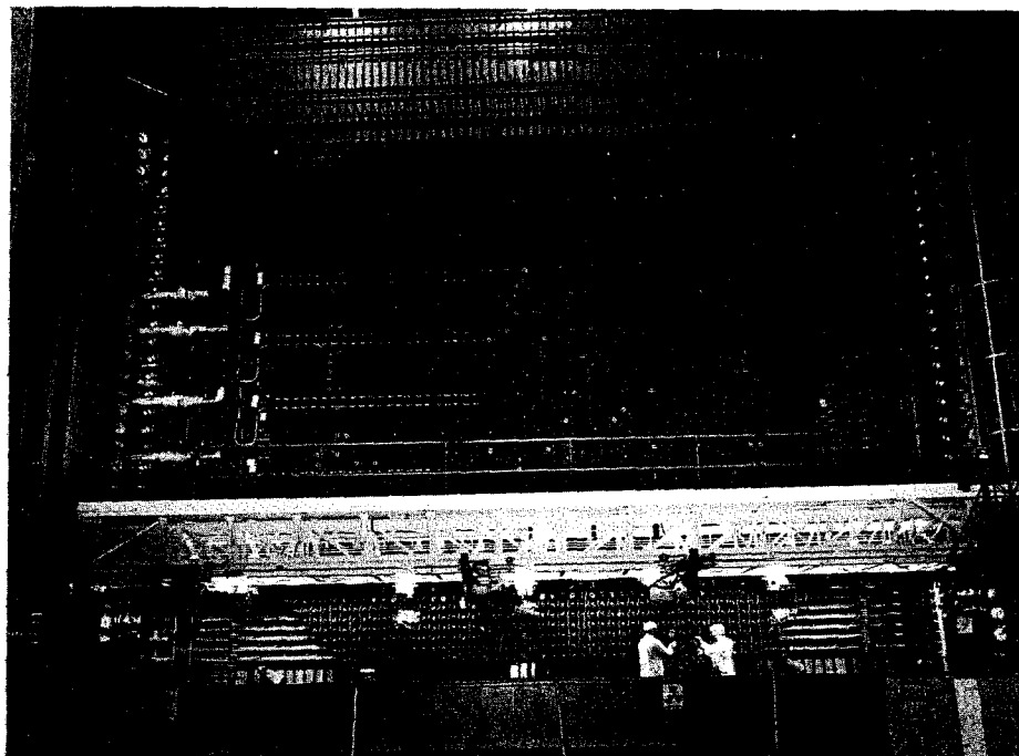
FIG. 11. Front face of a typical production reactor.
