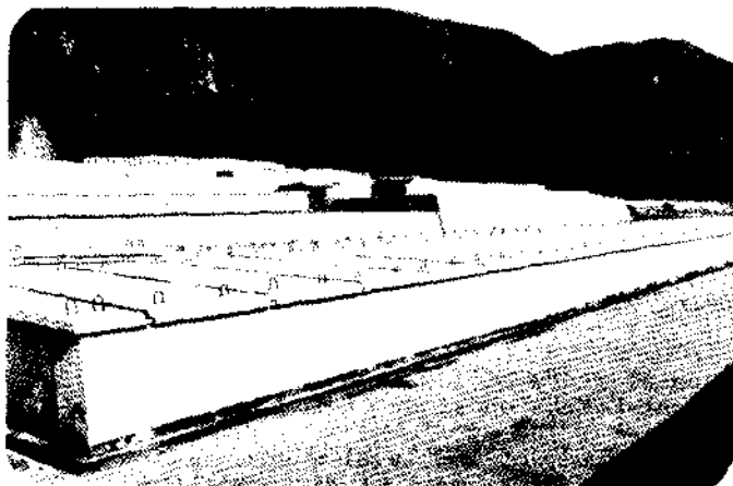
Fig. 3 Outside View of Concrete Trench
