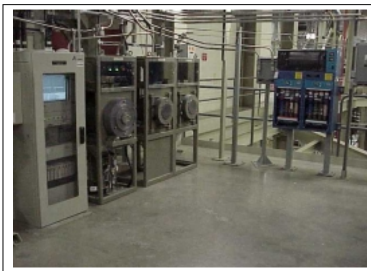
Fig.5 14 C Sampler Installed and Integrated With the Stack Monitoring System at Darlington Nuclear Plant
