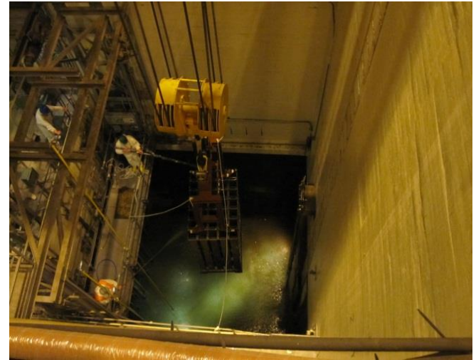
Racks removal (José Cabrera
