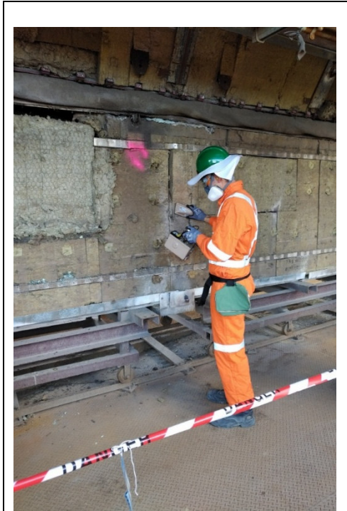
FIGURE 5-12: A TECHNICIAN CHECKING INSULATION TO DETERMINE ITS DISPOSAL PATHWAY.
