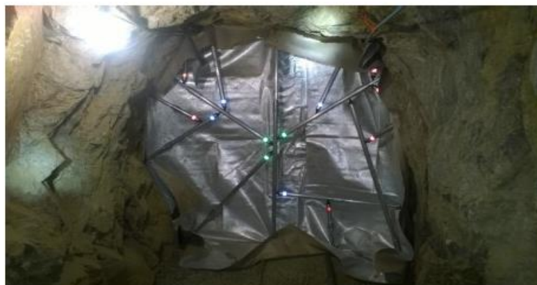
Fig. 1. Quick-Erect Stopping System (QESS) in the Edgar Mine, Idaho Springs, Colorado
