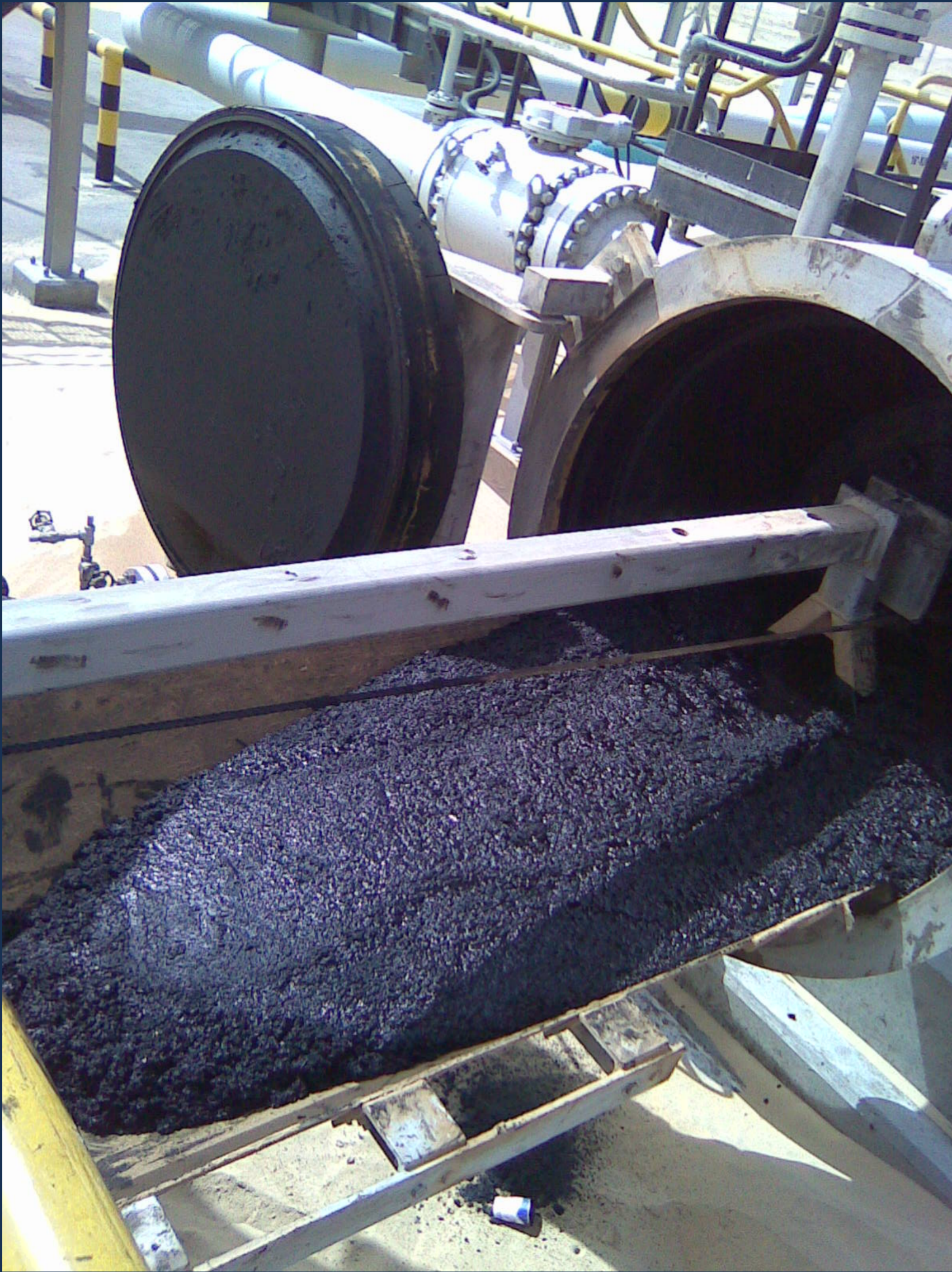
Fig.1. Black powder produced during pipeline scraping
