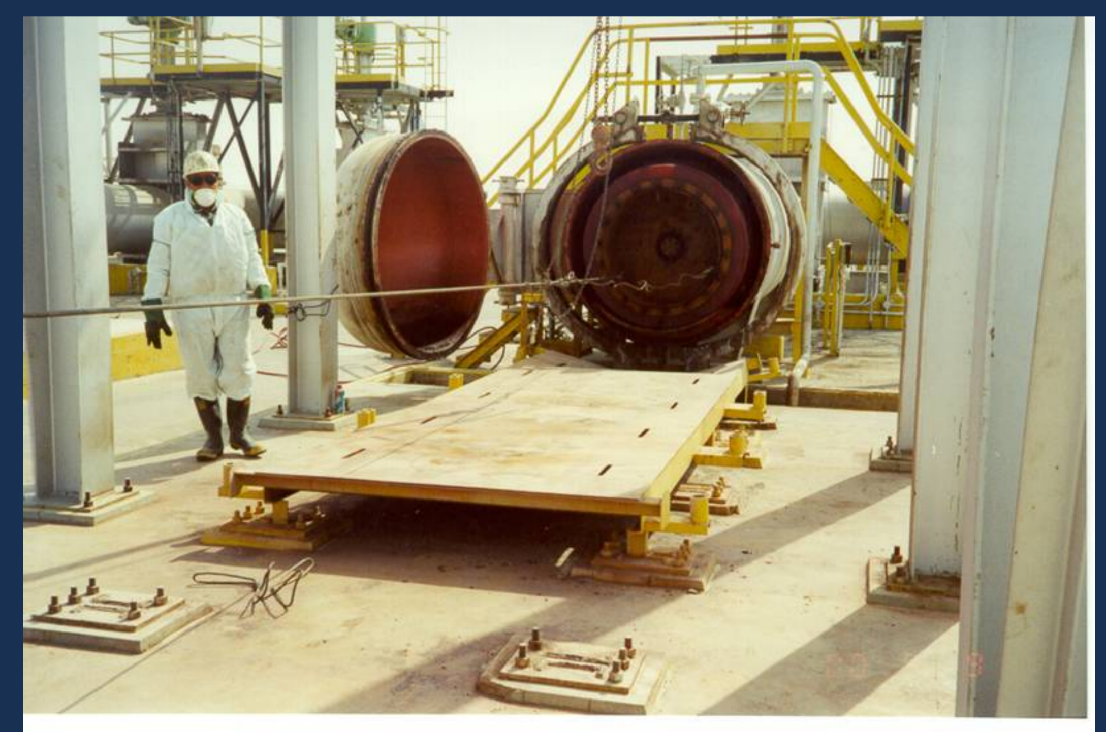
Fig.5. Worker recovering pipeline scraper
