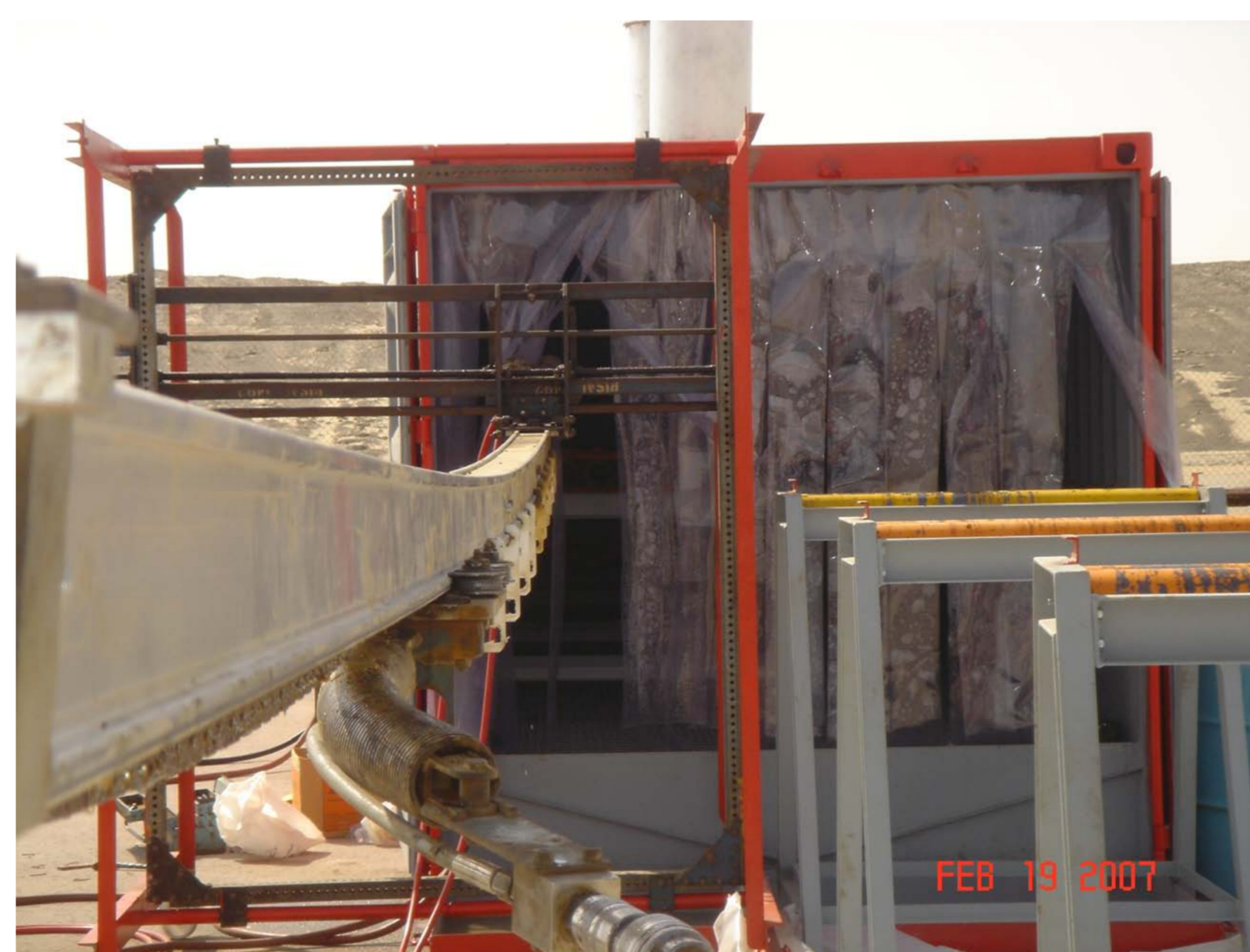
Fig.10. Lance delivering HPWJ is placed through tubular
