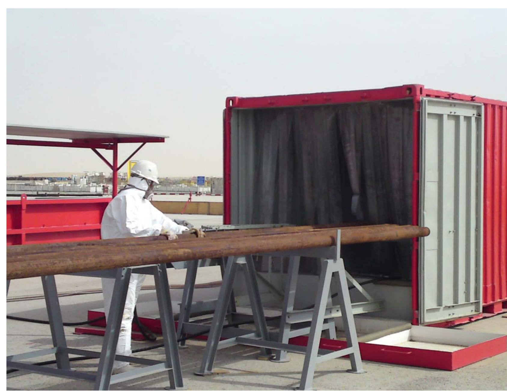
Fig.8. Tubular is placed in containment area
