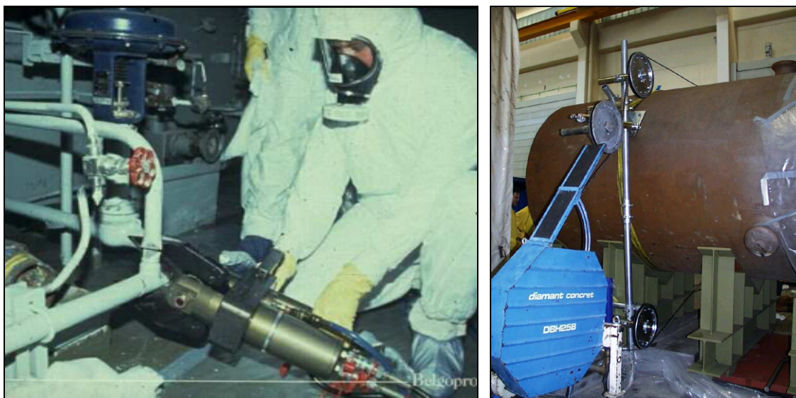
Figure 6. Examples for mechanical cutting techniques. Left: mechanical shears (BR3, Belgium), Right: diamond wire cutting for large components (HDB, Karlsruhe, Germany).
