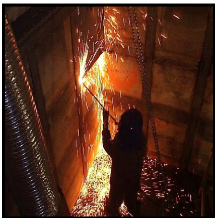
Fig. 5. and Fig. 6. Hot work to remove the Criticality Cell liner and pit
