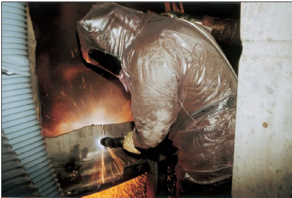
Figure 5. Examples for thermal cutting techniques. Plasma cutting.
