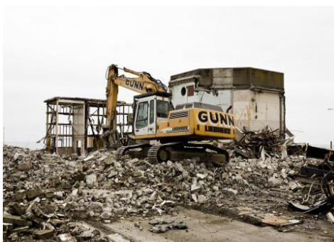
Fig. 7. Demolition of the Criticality Test Facility
