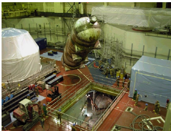
Fig. 4. Removal of a steam generator in Greifswald (KGR).
