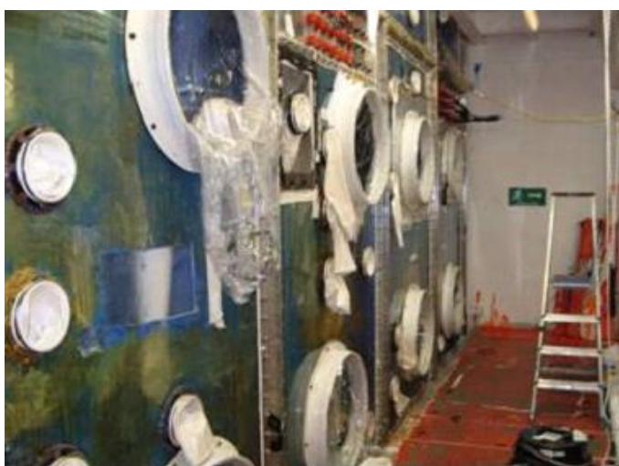
Fig. 14. Installed posting ports for the removal of glovebox internals
