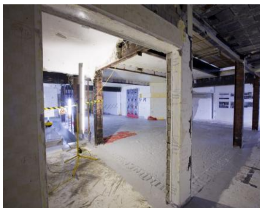
Fig. 4. Completed internal wall removal
