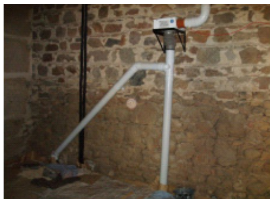
Fig. 8. Sub-floor piping installation for a sub-slab depressurization system in France (CSTB 2008).
