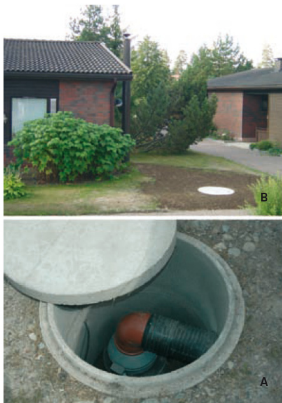
Fig 11. Exhaust fan in a well ring (A) and cover of the well ring as well as the exhaust pipe installed above the eave height of the building (STUK 2008).
