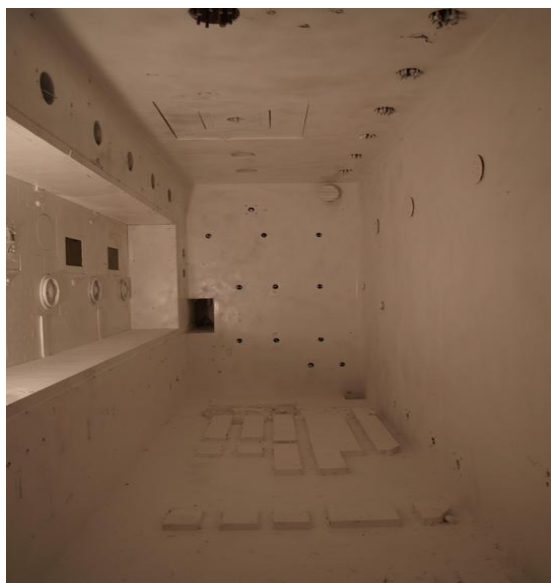
Fig. 2. Peelable paint applied.
