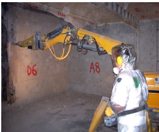
Fig. 3. Demolition of internal walls with a Brokk
