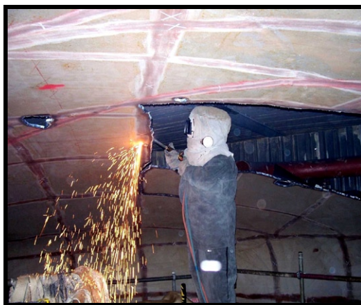
Fig. 5. and Fig. 6. Hot work to remove the Criticality Cell liner and pit
