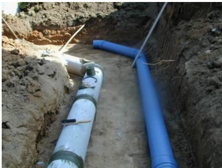
Figure 5: Installation of concrete and plastic earth tubes in the ground
