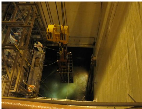
Racks removal (José Cabrera)
