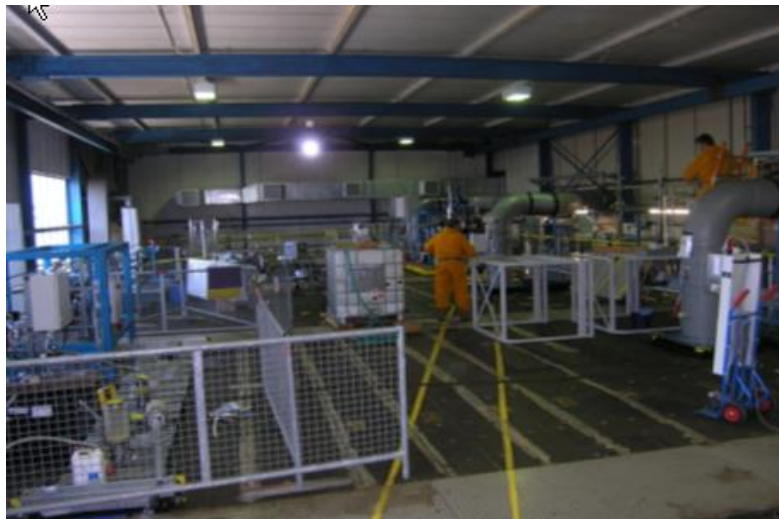
Figure 4 'High' Level Activity (HLA) tank tops
