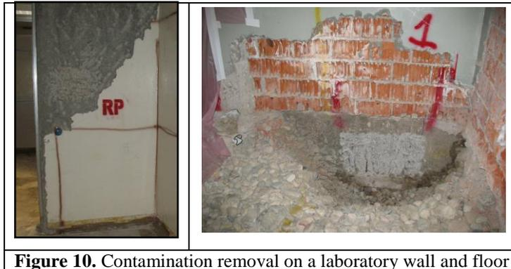
**Figure 10.** Contamination removal on a laboratory wall and floor
